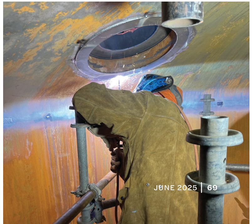
Lands is shown making a sulfuric acid tank repair.
