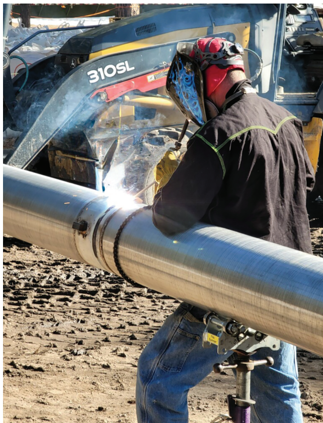
Lands performs SMAW on a stainless steel casing run for a water well pipe.
